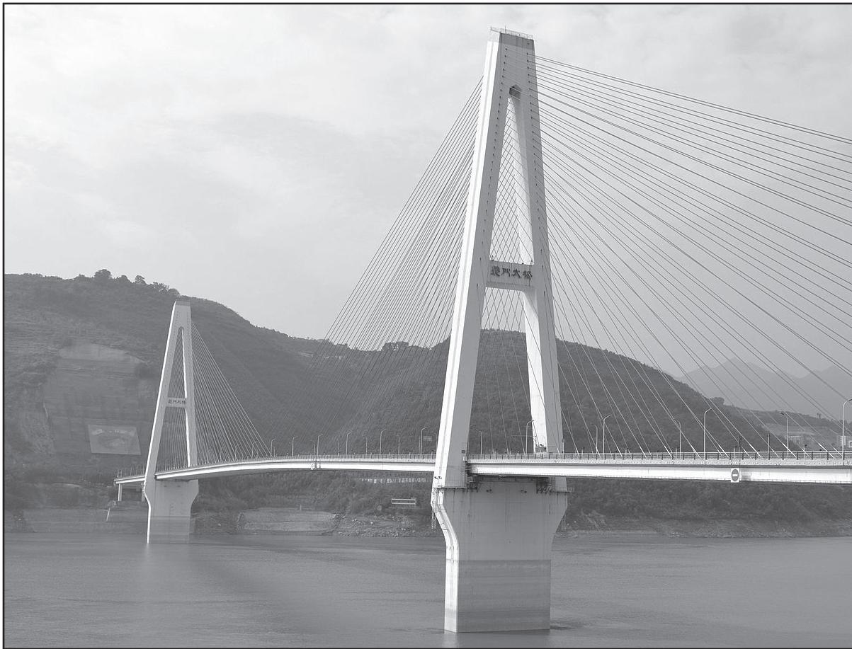
The Fengjie Yangtze Bridge is a cable-stayed bridge which crosses the Yangtze River in Fengjie, Chongqing, China. Completed in 2005, it carries 4 lanes of traffic. (Photo: Wikimedia Commons)
